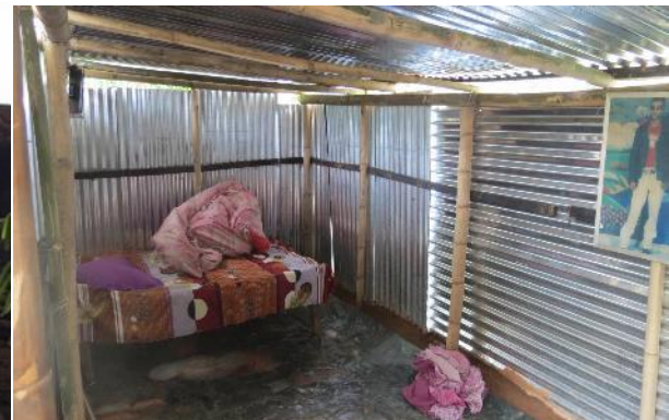
Temporary Shed built with Foundation help
